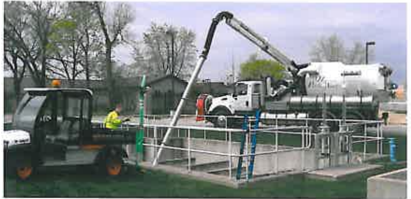
Crews clean the Chlorine Contact Tanks as part of maintenance
