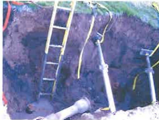
Repairs at Lake Shore & Sunnyside
