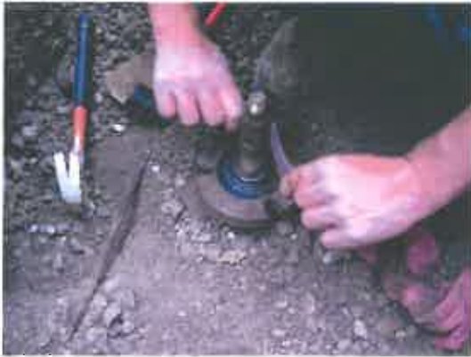
Preparing for a New Packing Gland
