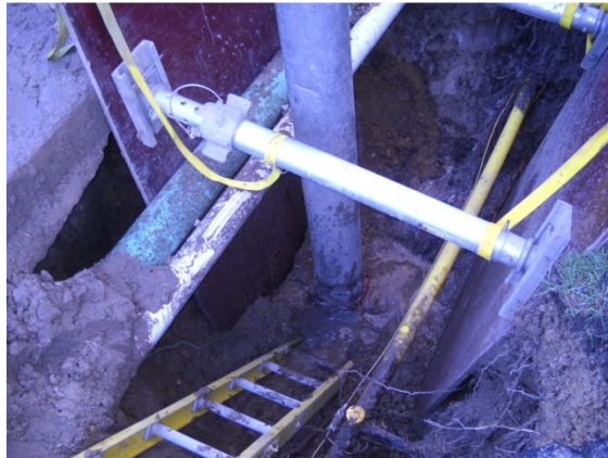
Tight Quarters Excavated by Vac Truck
