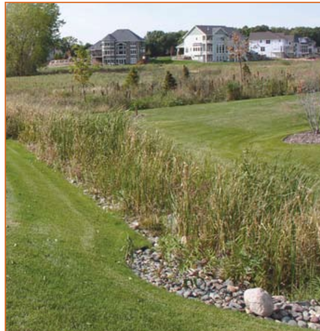
A road ditch can serve as a bioswale. The rock trench and wetland vegetation are notable features along with the natural drainageway in the background that serves as a bioswale for residential runoff.
